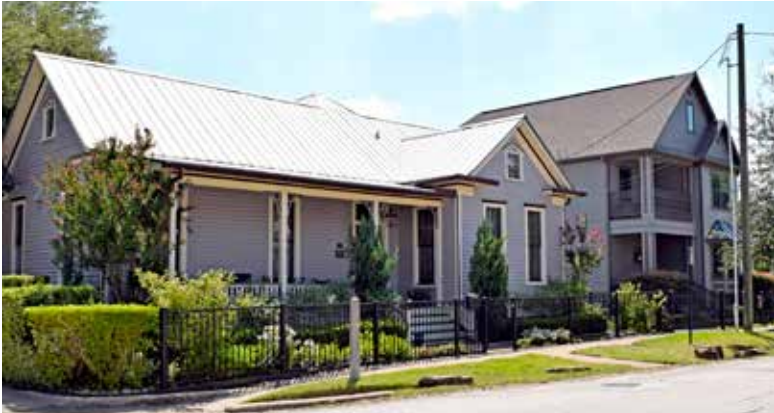
Site design considers street frontage, building setbacks, parking, signage, service and utilities, fencing and screen walls. Shallow front yards, continuous planting strip, and fences are site features noted in this image.
