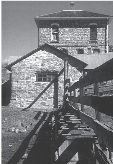
Fence detail at the Frawley Ranch
