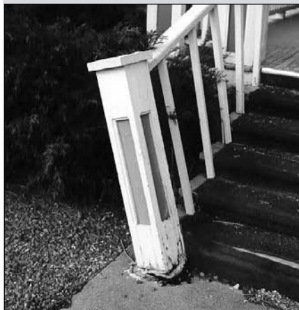
Before: A deteriorated handrail
