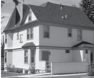
Accessibility ramp added to 1002 N. Weber during technical rehabilitation.
