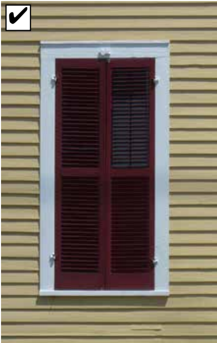
Shutters should be real, operable units and should be correctly proportioned to the window opening.
