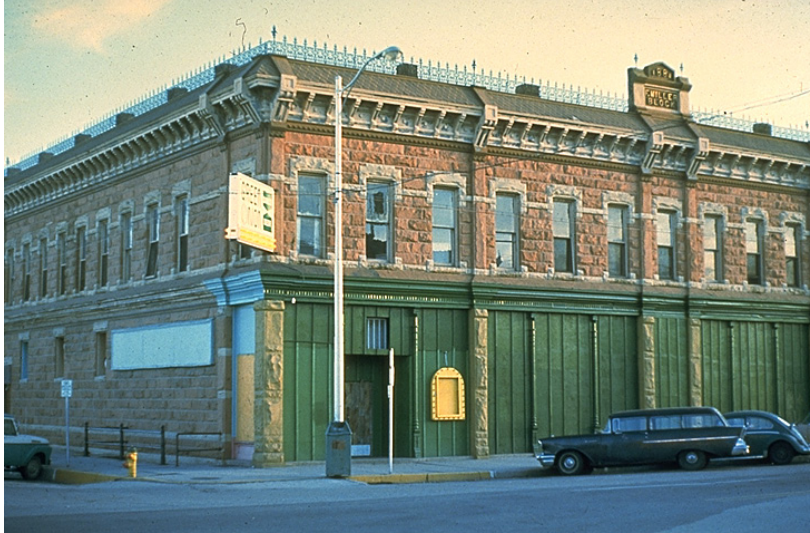
Before: In the early 1980s, the windows in the Miller block were boarded and architectural details needed repair.
