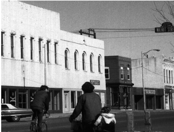
Reed and Dauthe building, before.
