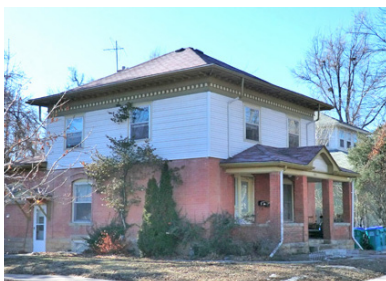
A strong historic context exists in much of the Eastside and Westside neighborhoods.
