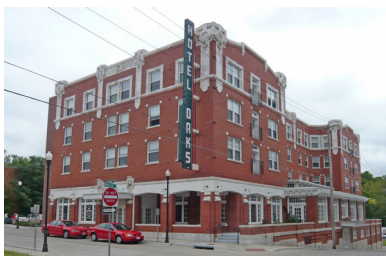
Hotel renovations, such as the Hotel Oaks, are models for future preservation projects.
