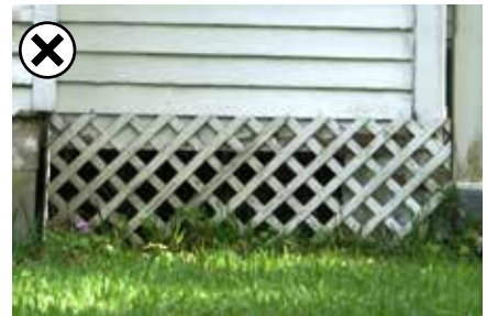
Examples of inappropriate unframed lattice
