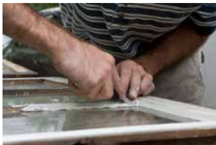
Replacing glazing putty © iStockPhoto.com/Elaine Odell
