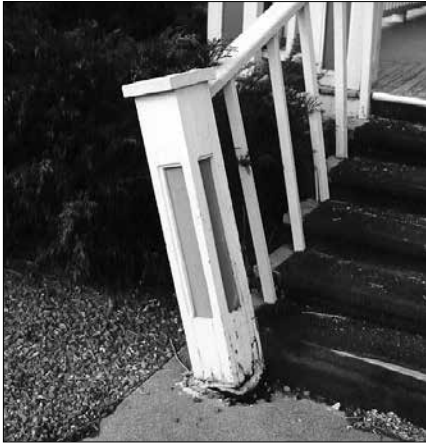
Before: A deteriorated post and handrail
