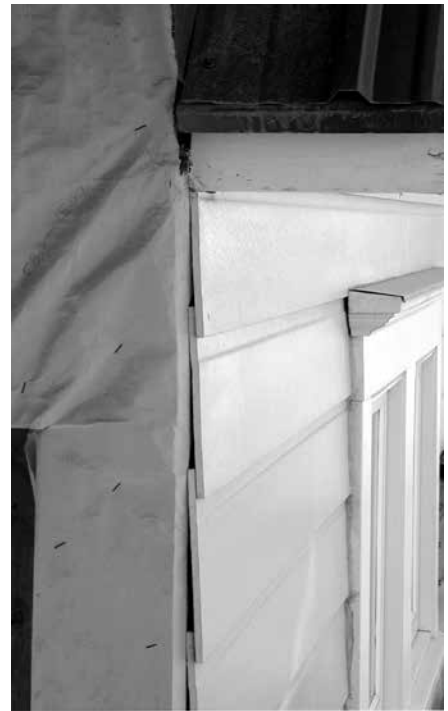
Installation of fiber-cement siding
