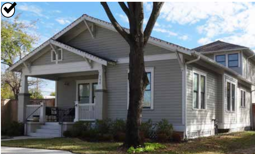
The walls of this appropriate two-story rear addition are inset from the historic building, so that the original rear corners remain visible. The side wall addition is small and preserves the original eave line. Also, the hip roof on the addition reduces its scale and makes it more compatible with the historic building.
