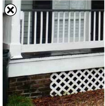
Screening panels may be installed between foundation piers. Screening panels should be framed around the lattice pieces.
