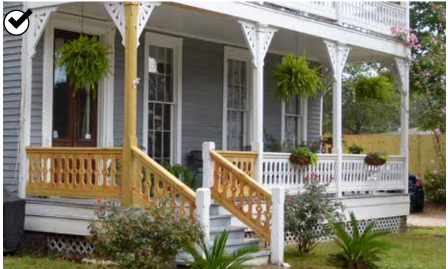
Replacement porch elements (unpainted) match the original components.
