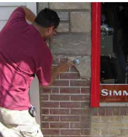
3. Restoration to a previous period by removal of "stone" paneling
