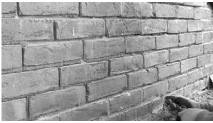
Repoint mortar joints where there is evidence of deterioration.
