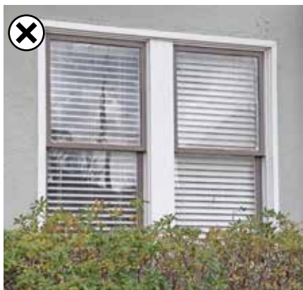
Much of the window appears to be repaired except the trim has been replaced. The thin trim and mitered corners are inappropriate and should have matched the original detail.
