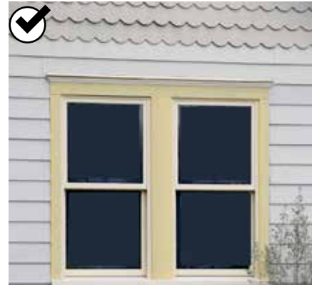
The use of cementitious siding and a contemporary detail in the gable are ways in which to differentiate an addition to a historic building.
