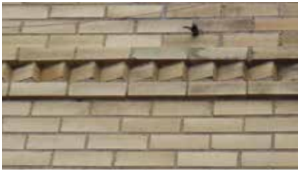
Repoint mortar joints where there is evidence of deterioration.
