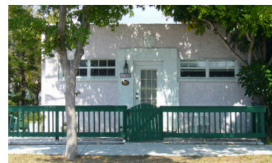
West Palm Beach is seeking to protect its unique architectural heritage.
