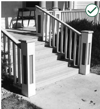
After: Railing has been repaired and the base of the post has been replaced in-kind. This is an appropriate approach.
