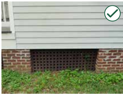
Preserve the original piers, foundation and foundation infill whenever possible.
