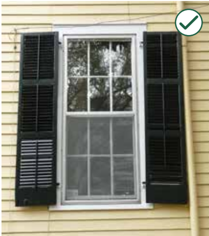
Size a new shutter to precisely fit the window opening. The shutters above are inappropriate.
