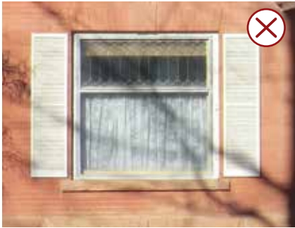
Size a new shutter to precisely fit the window opening. The shutters above are inappropriate.
