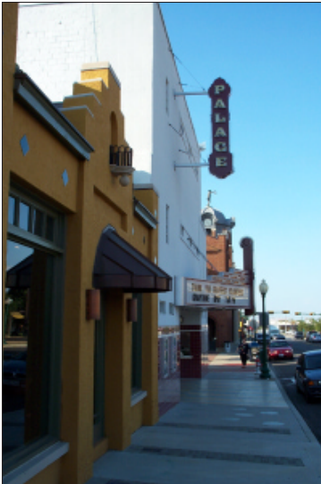
The restoration of the historic Palace Theater has been a preservation success story for downtown Grapevine.
