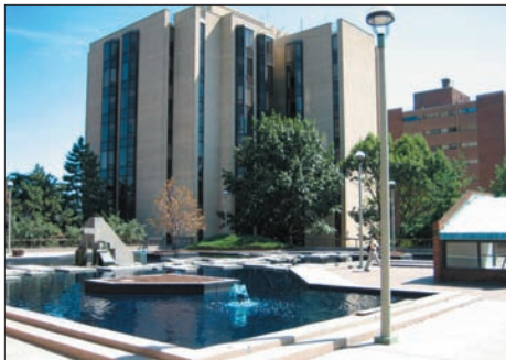
Clerc Hall at Gallaudet University in Washington, D.C. is a deaf student housing renovation project being undertaken by Winter & Company's Special Needs Studio.
