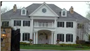
Newly constructed homes are significantly larger in scale.
