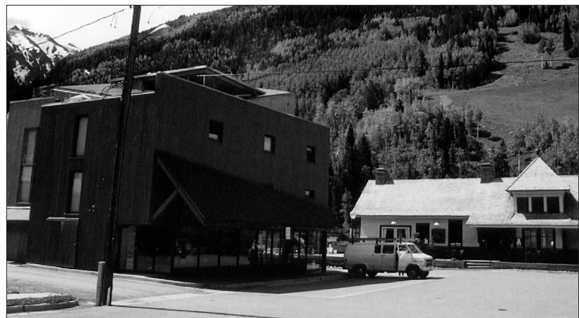
The depot after renovation, with a new contemporary infill project in the
