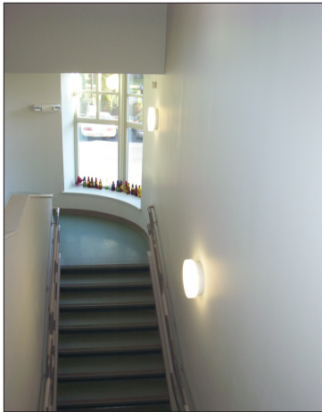
Stairway from Second Floor
