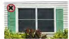
Do not install shutters that are narrower than the associated window or opening.
