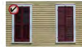
Match the width of new or replacement shutters to the width of the associated window or opening.
