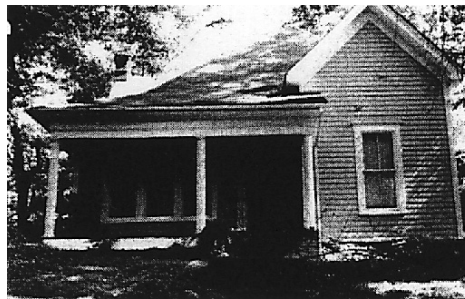
This house exhibits the offset porch that often accompanies an L-Plan house. The horizontal lap siding is also a typical feature.
