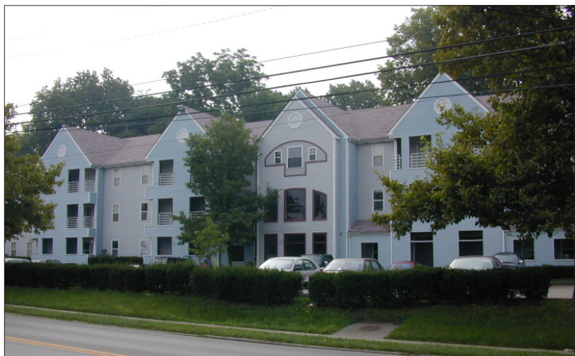
Existing infill development was perceived as missing some of the essential design features seen traditionally in pedestrian-oriented neighborhoods. In this case, parking separated building entrances from the sidewalk edge.
