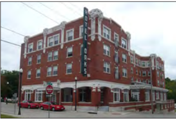
Hotel renovations, such as the Hotel Oaks, are models for future preservation projects.
