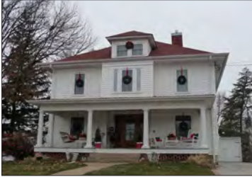
Many doctors moved to town to set up practice near the mineral springs and lived in the historic residences.
